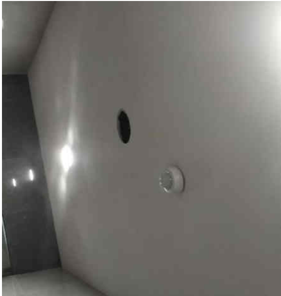
Sensor based Bulbs in washroom
